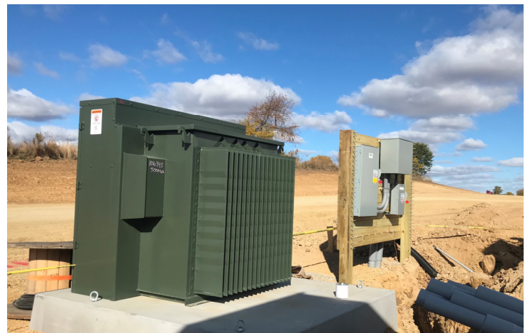
Temp Power Setup Complete – Waiting on Inspection
