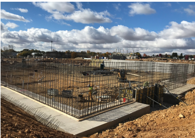
Rebar Tying & Pouring Gym Retaining Wall
