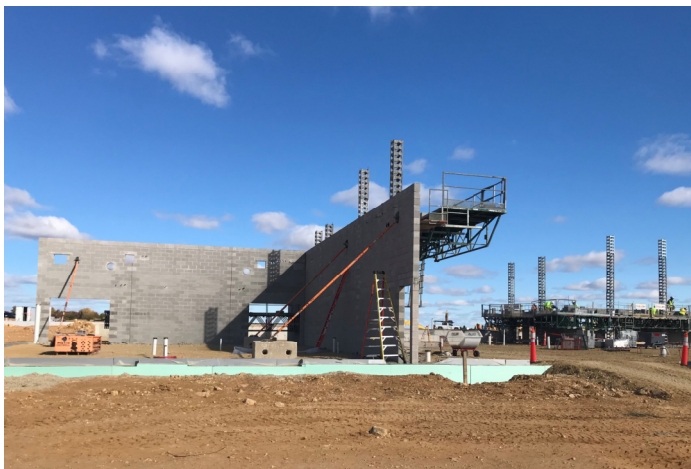
Interior CMU Walls Going Up in Area C and D
