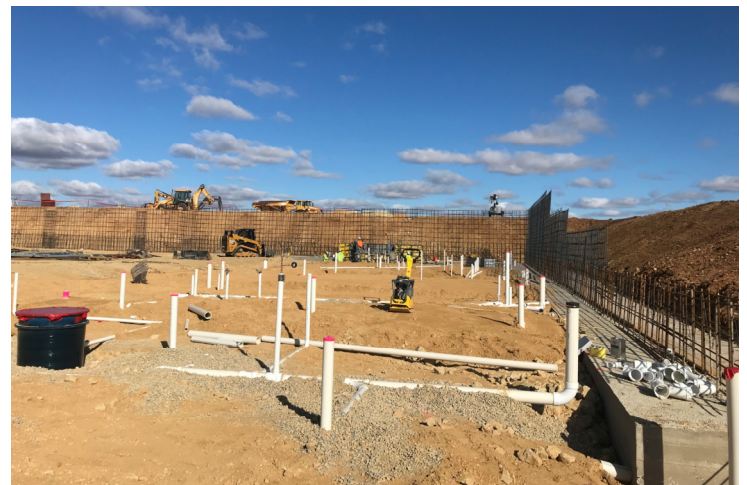
Gym Plumbing Rough-ins
